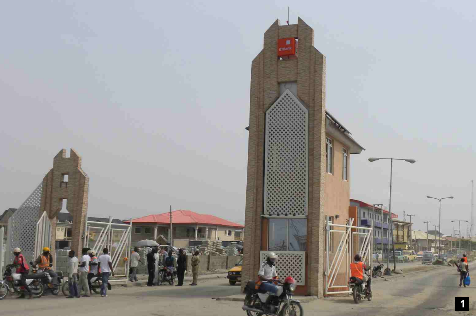
1. Lekki Peninsula Phase One 2nd Gate "The Beacon"
