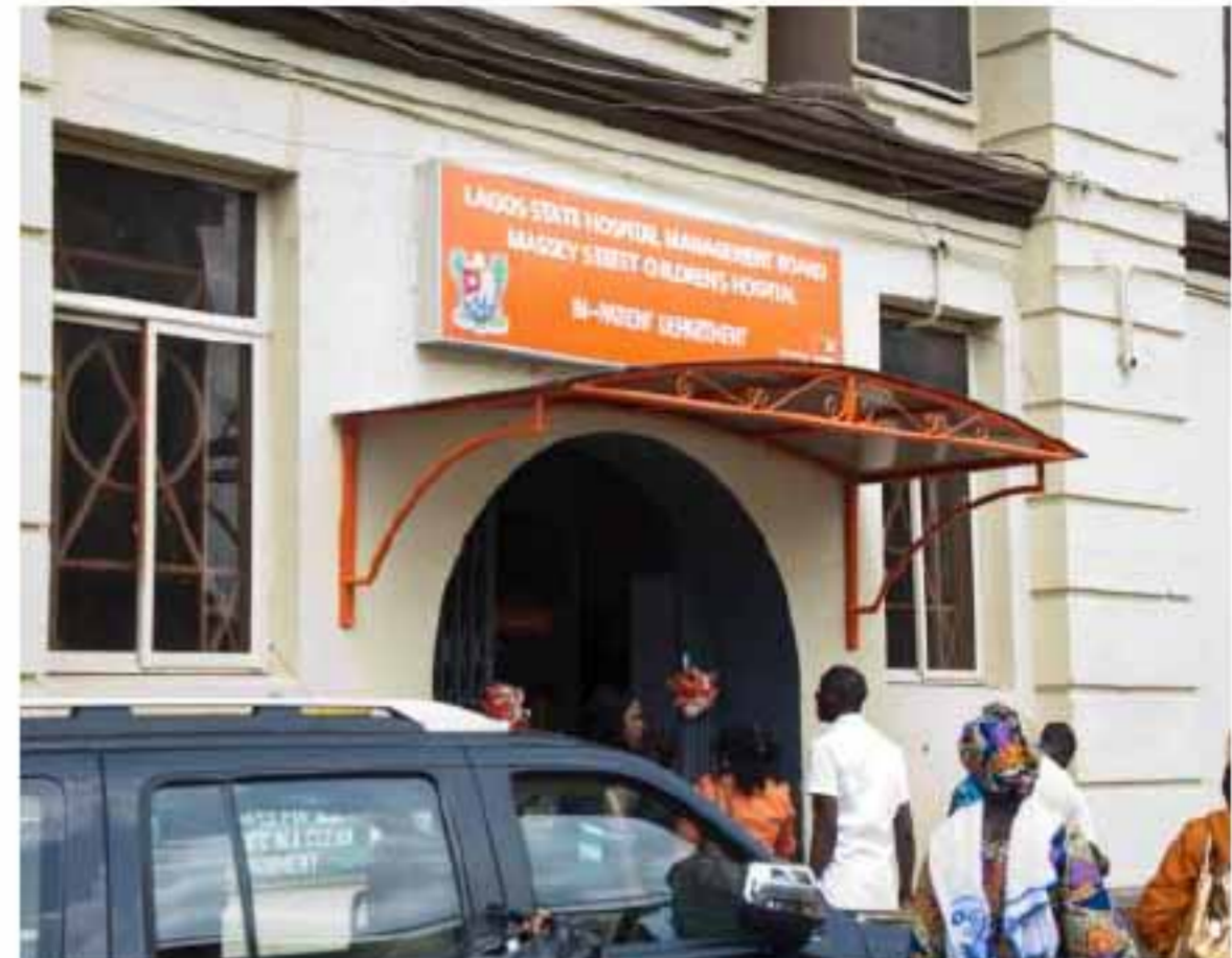
Massey Street Children's Hospital. Before and after the renovations.
